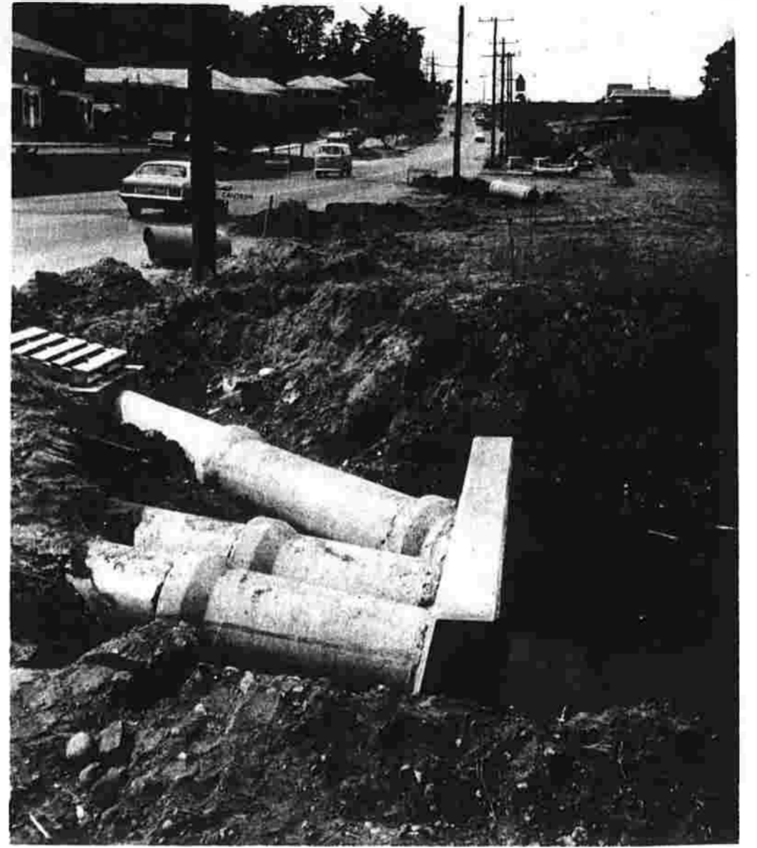
Storm sewer installed
